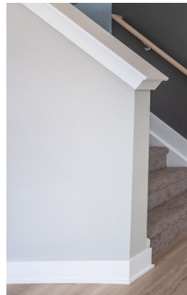
1/2 Wall Railing Oak cap painted or stained
